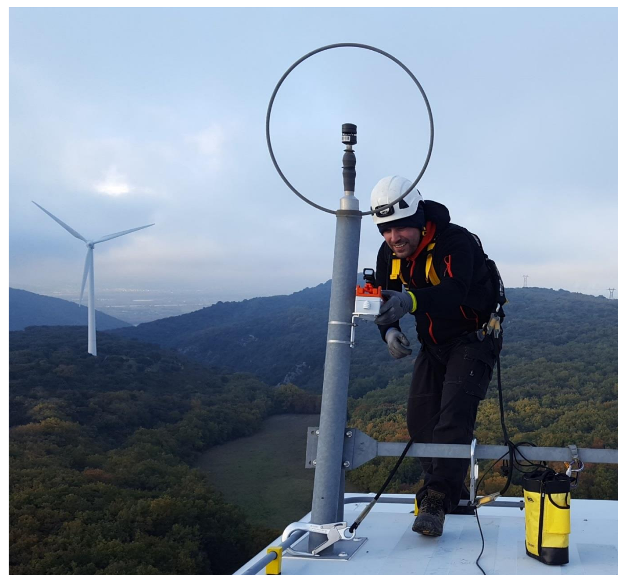
Figure 1: Windfit box set on the met mast of a Vestas V66 of the Roussas-Claves wind farm by RES
